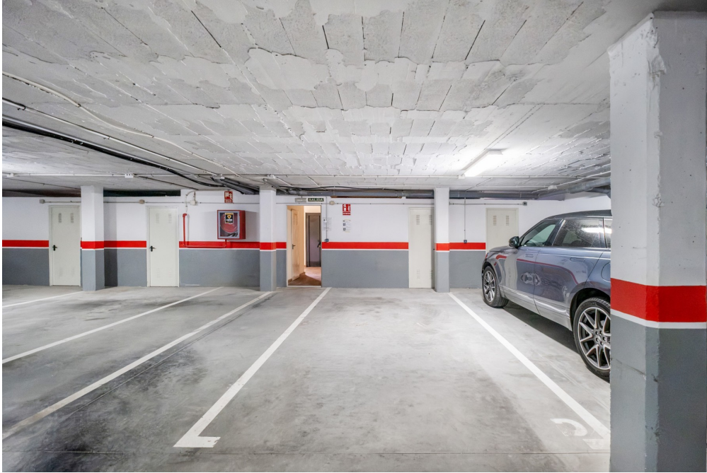
Underground garage in the apartment building
