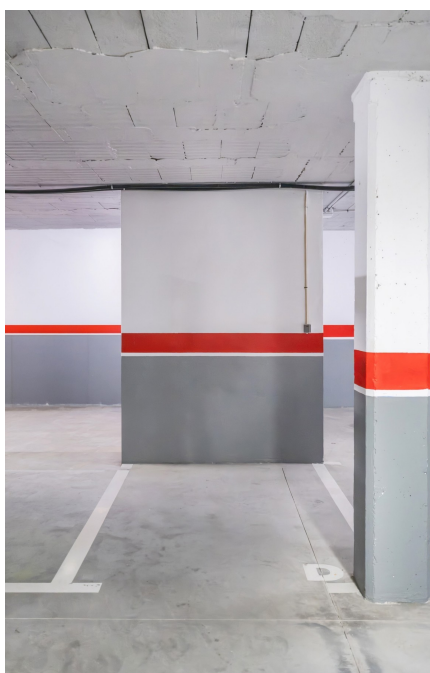
Private parking space in the garage
