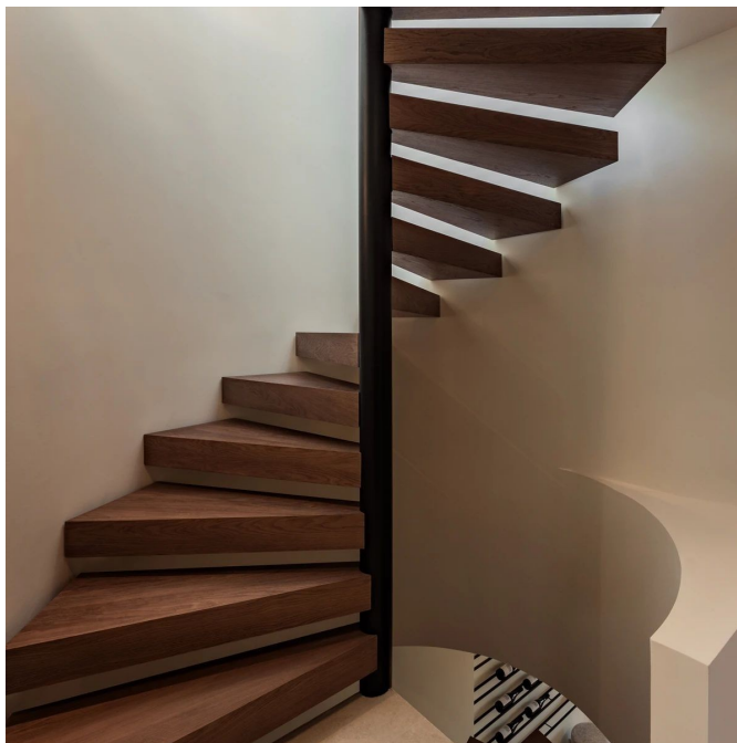
Floating timber staircase
