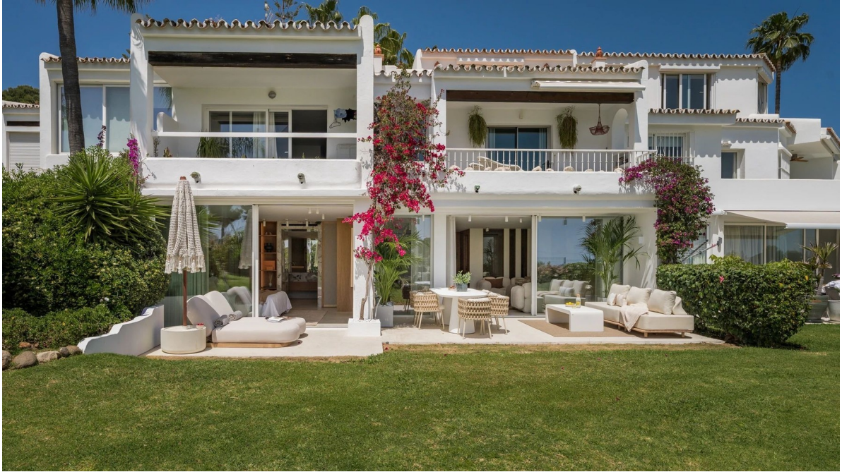
Garden facade with bougainvillea and terrace
