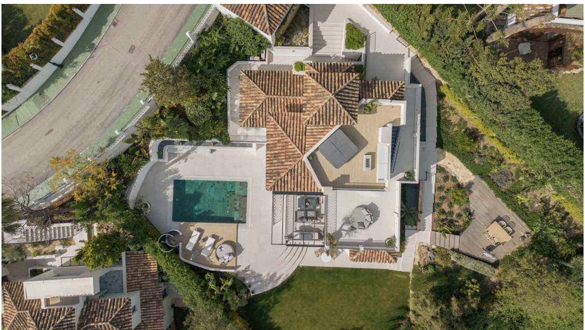
Aerial view of the villa plot and surrounding neighbourhood
